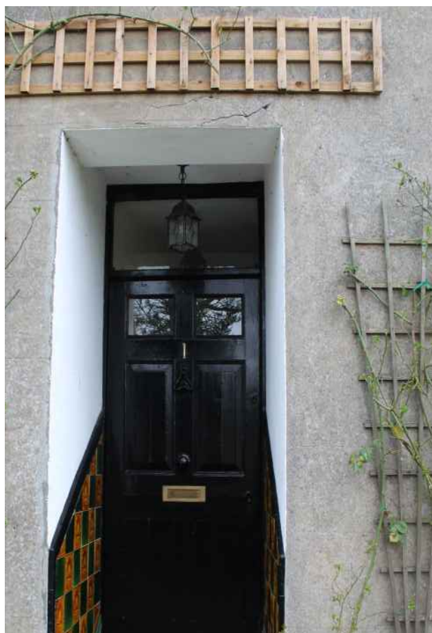
Figure 106 Decorative tiles at Number 1, Mistley Green
