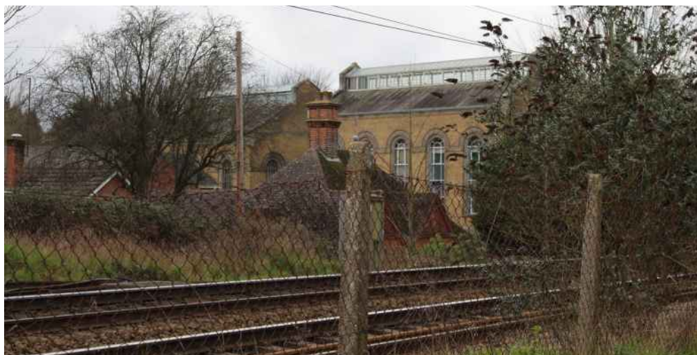
Figure 69 Pump House and railway, Lawford Water Works
