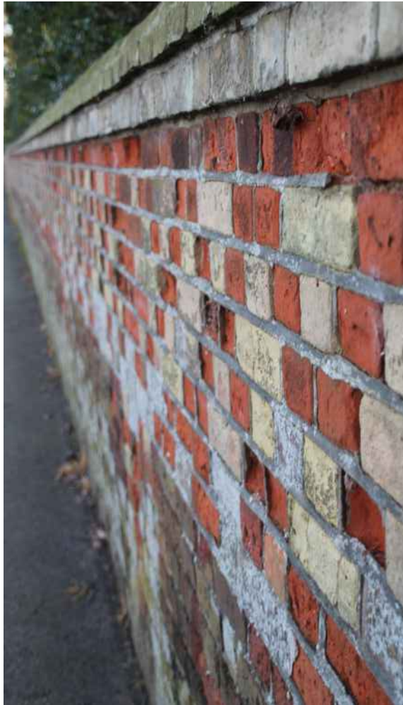
Figure 158 Mistley Place Park historic wall
