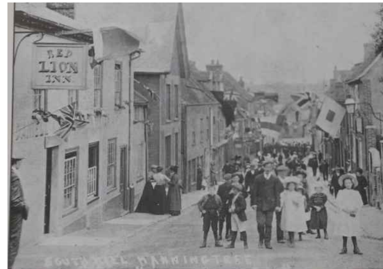
Figure 8 South Street, Manningtree c.1900-1925
