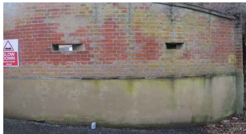
Figure 72 Boundary wall with loop holes, Lawford Water Works
