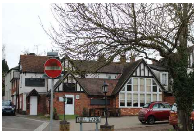
Figure 21 The Swan, Brook Street
