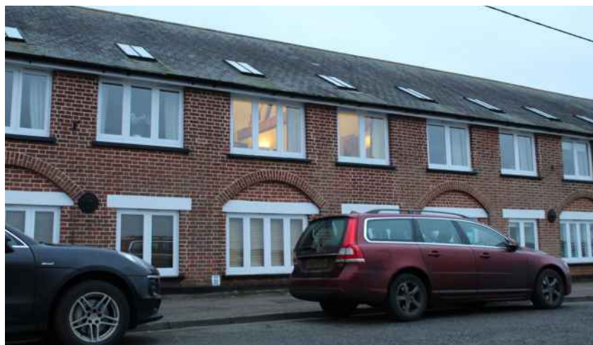
Figure 76 1-10 Brooks Malting with partially infilled arches
