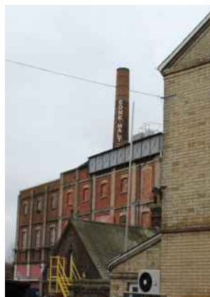
Figure 119 EDM Chimney from Mistley High Street along with maltings building South east of EDM
