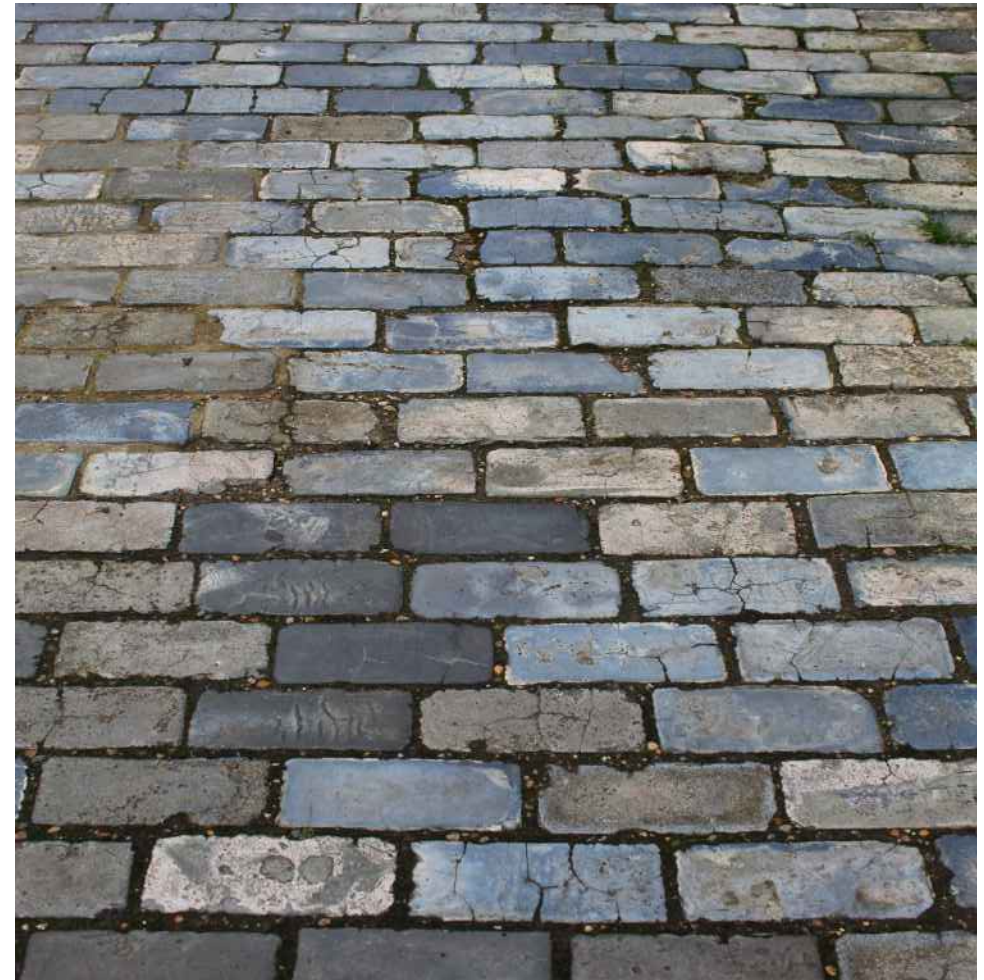
Figure 161 Historic Scoria brick paving detailing
