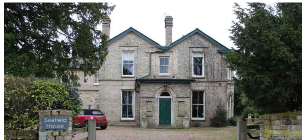
Figure 123 Seafeld House (The Elms)
