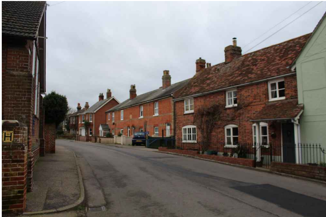
Figure 62 View south along Trinity Road
