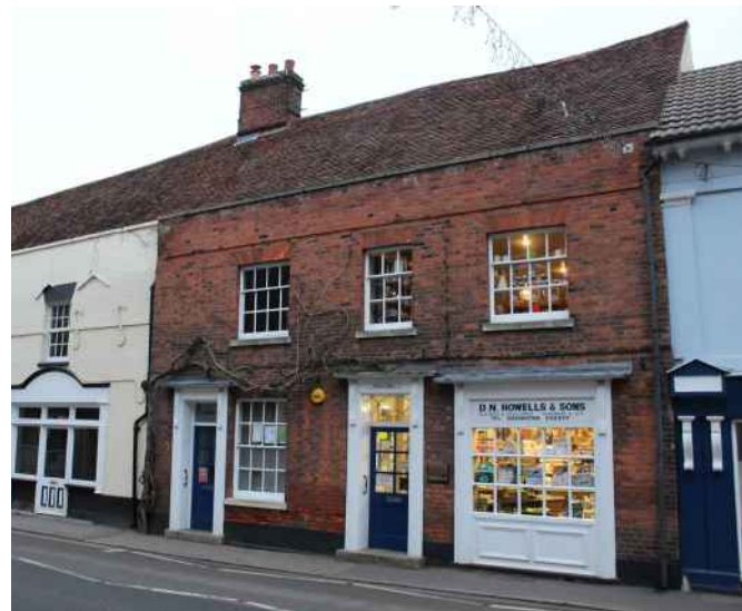
Figure 148 Historic shop frontage, Manningtree
