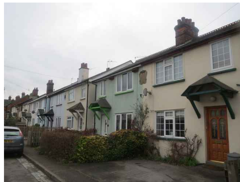
Figure 151 Lack of boundary treatments along California Road
