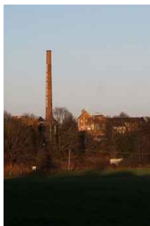
Figure 120 EDM Chimney from Green Lane
