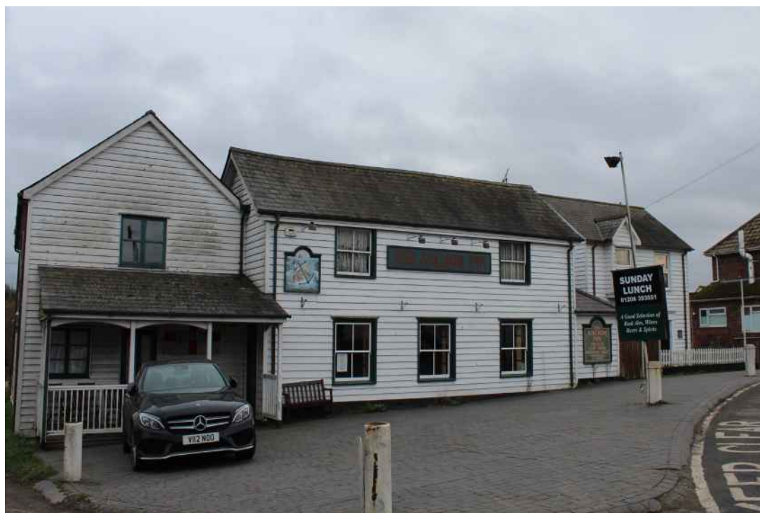
Figure 127 The Anchor Inn, Harwich Road
