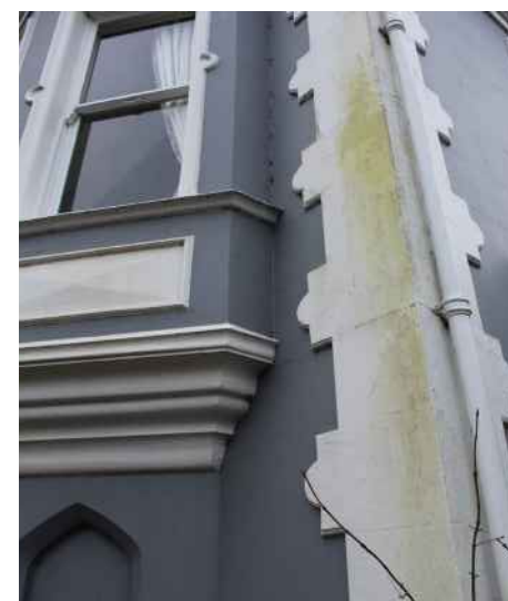
Figure 100 Buckle quoin detailing, Mistley House
