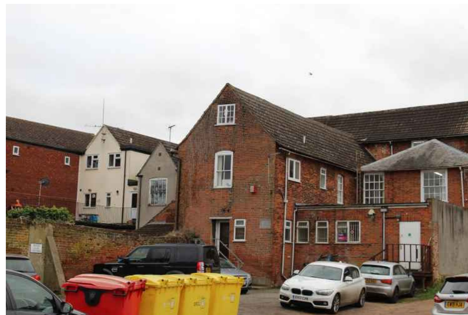
Figure 145 Parking for residents and businesses, North Street
