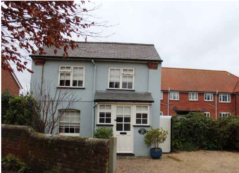
Figure 68 Barnfield Cottage, Barnfield
