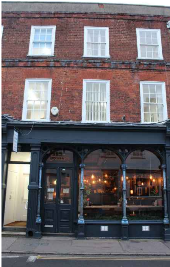
Figure 147 Historic shop frontage, Manningtree
