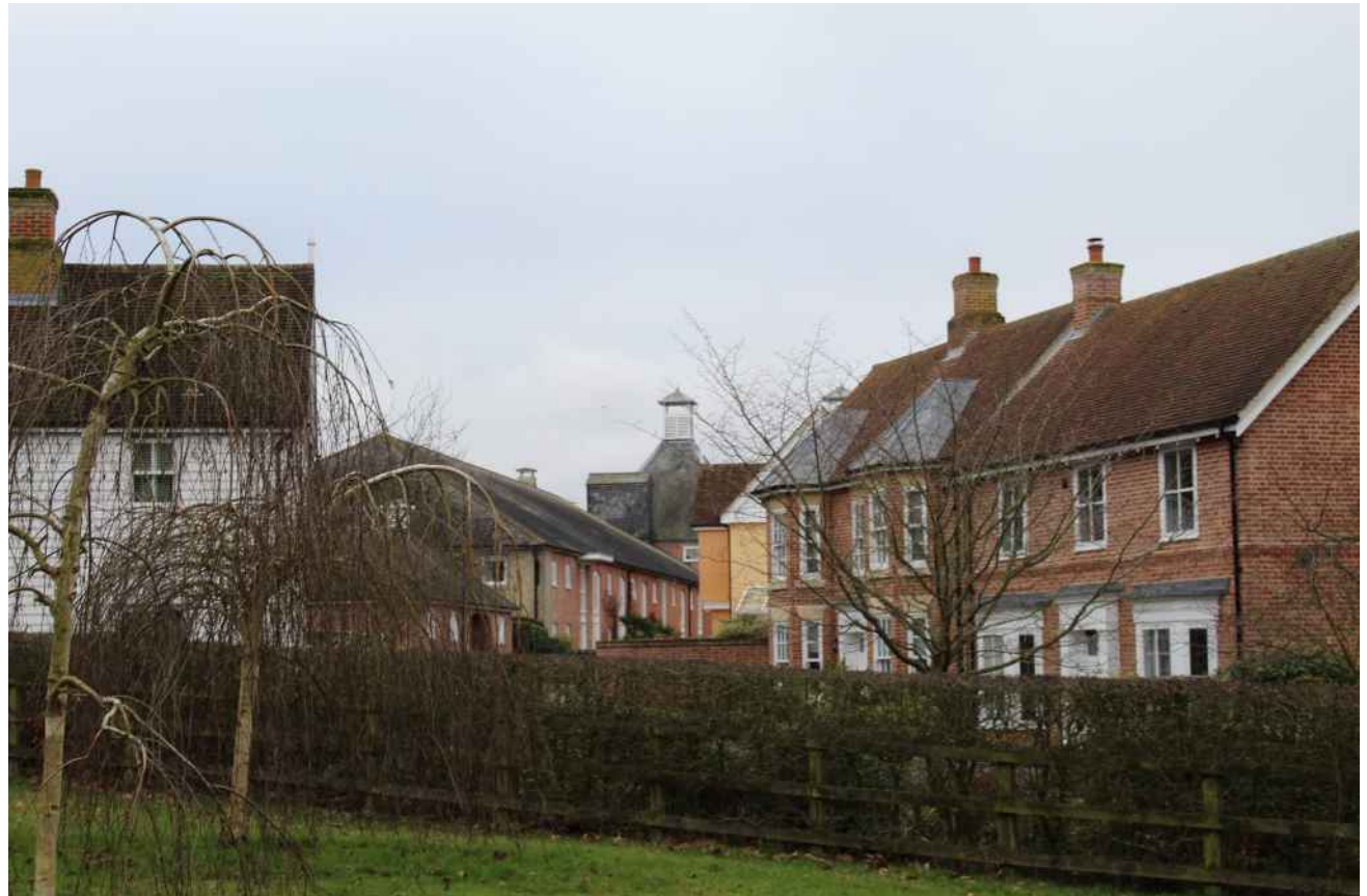
Figure 74 Listed maltings buildings at centre of development
