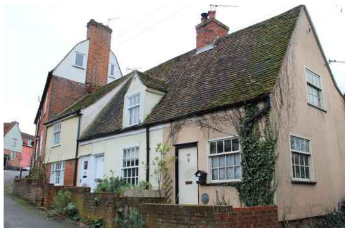
Figure 45 Listed cottages along Brook Street
