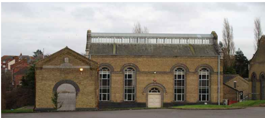
Figure 70 Pump House, Lawford Water Works
