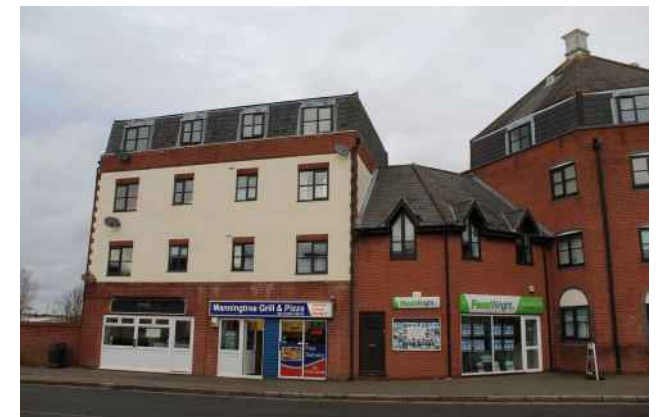
Figure 58 Blue brick window heads and sills
