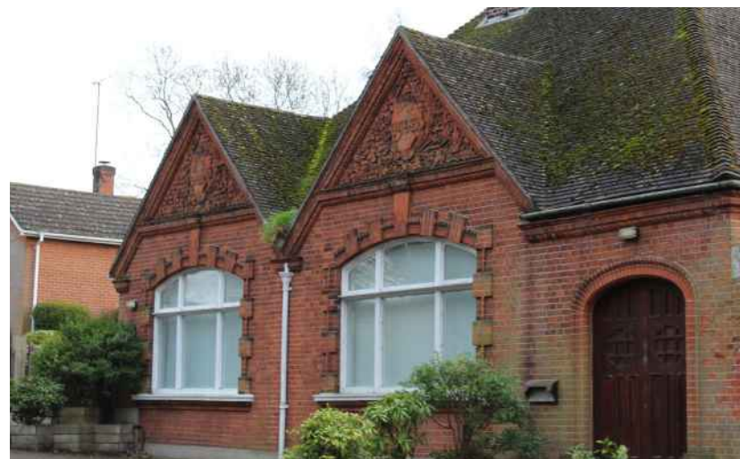
Figure 71 The Bungalow, Lawford Water Works
