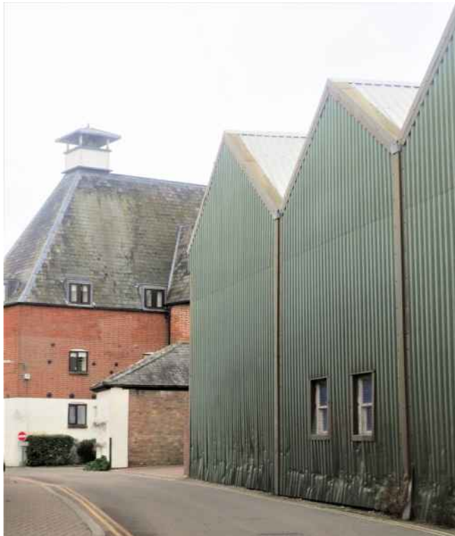
Figure 35 Maltings Kiln and Jewsons warehouse
